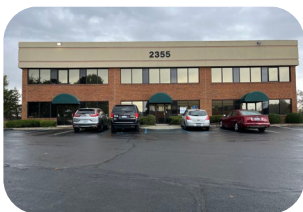
Huguenard Drive office building
